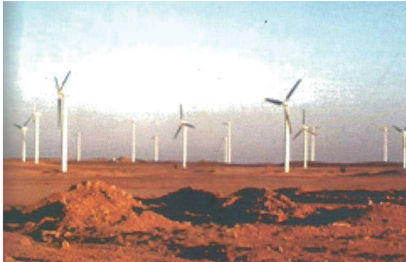
Figure (5) Wind Farms at Zafarana
